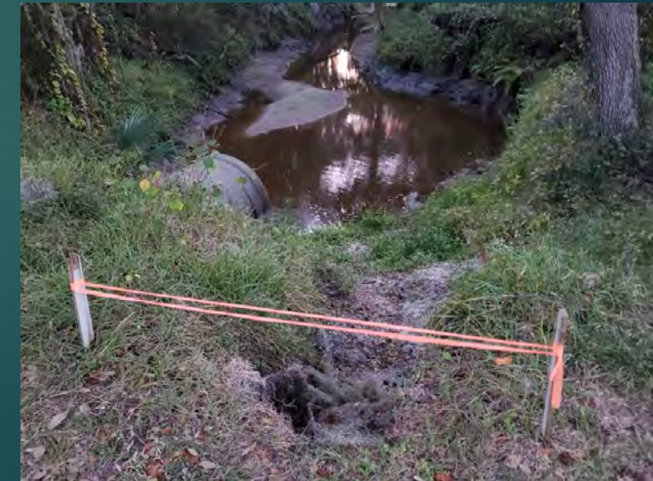
Erosion at Creek drainage culvert
